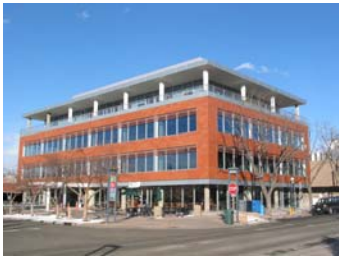
Renovation of 200 Fillmore Street Denver, Colorado
